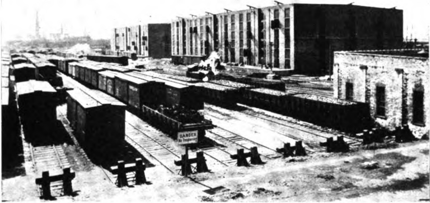
A Portion of the Union Freight Depot on the Bush Plant
